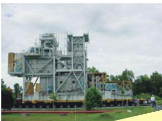
transporting and installing two turbo compressors, each weighing 300 MT with dimensions of 27 M length, 15.50 M height and 7.15 M width, was due to meticulous planning and stringent safety precautions and procedures.
